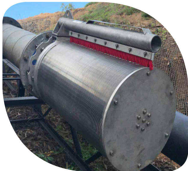
Self cleaning fish screen attached to a pump site. Photo: Craig Boys
