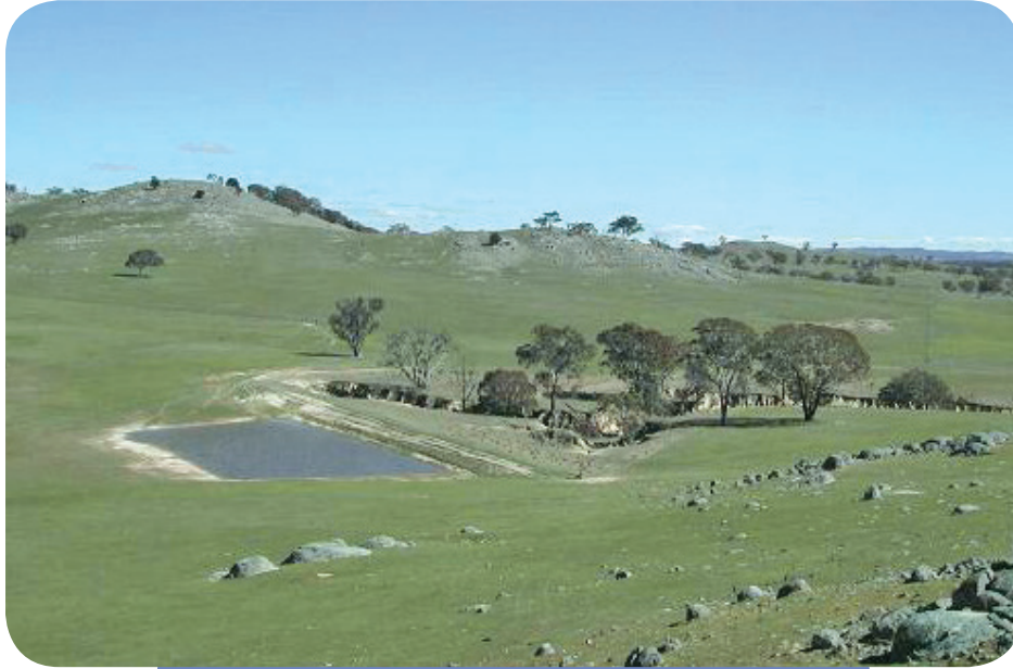
Gully control structure (dam) built above gully head.
