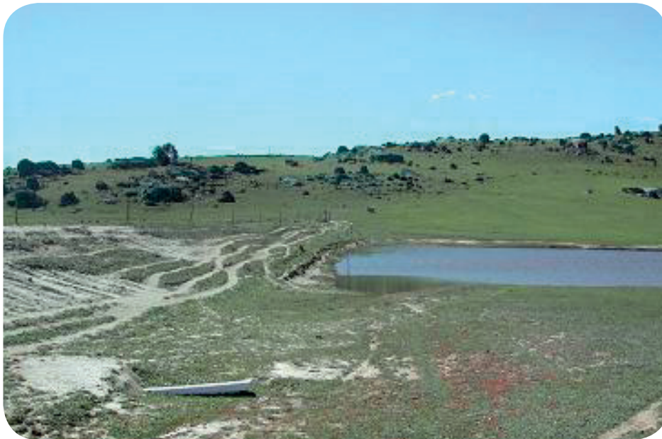
Pipe through bank of gully control structure (dam) to reduce the frequency of flow through primary spillway. This helps to prevent the spillway becoming sodden and prone to erosion.
