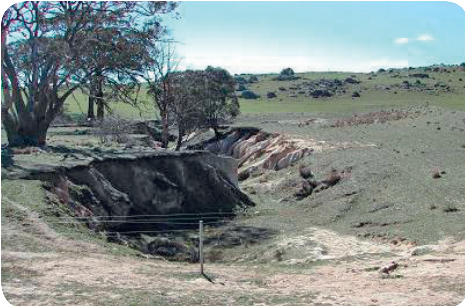
View of gully below gully control structure.
