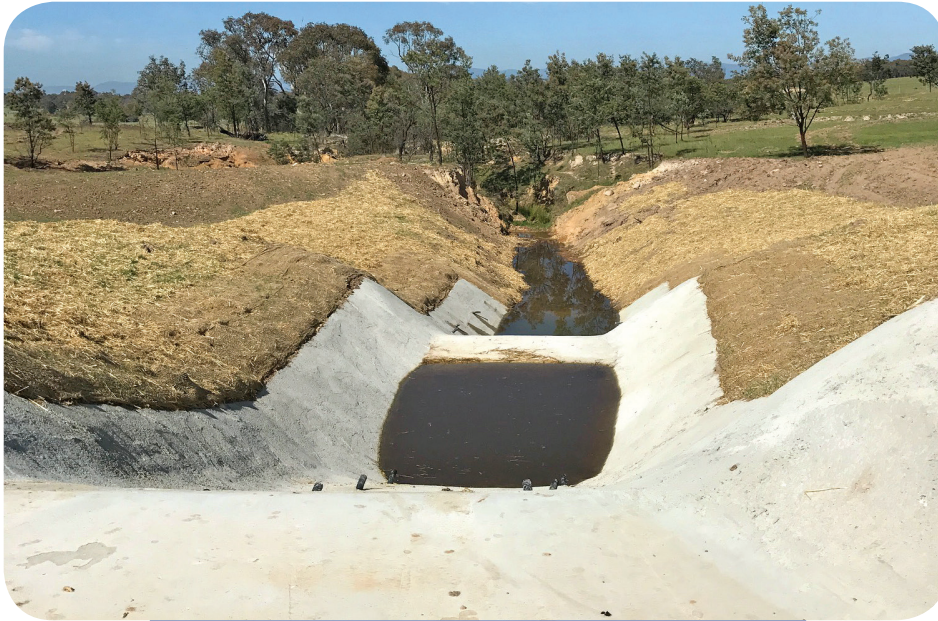
Concrete flume: directing flow into stilling pond.
