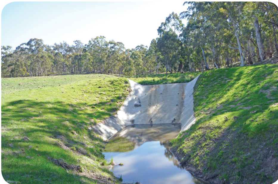
Concrete flume well vegetated.
